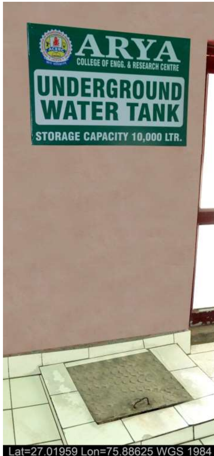
Underground Tank 1: Capacity 10,000 Ltr.
