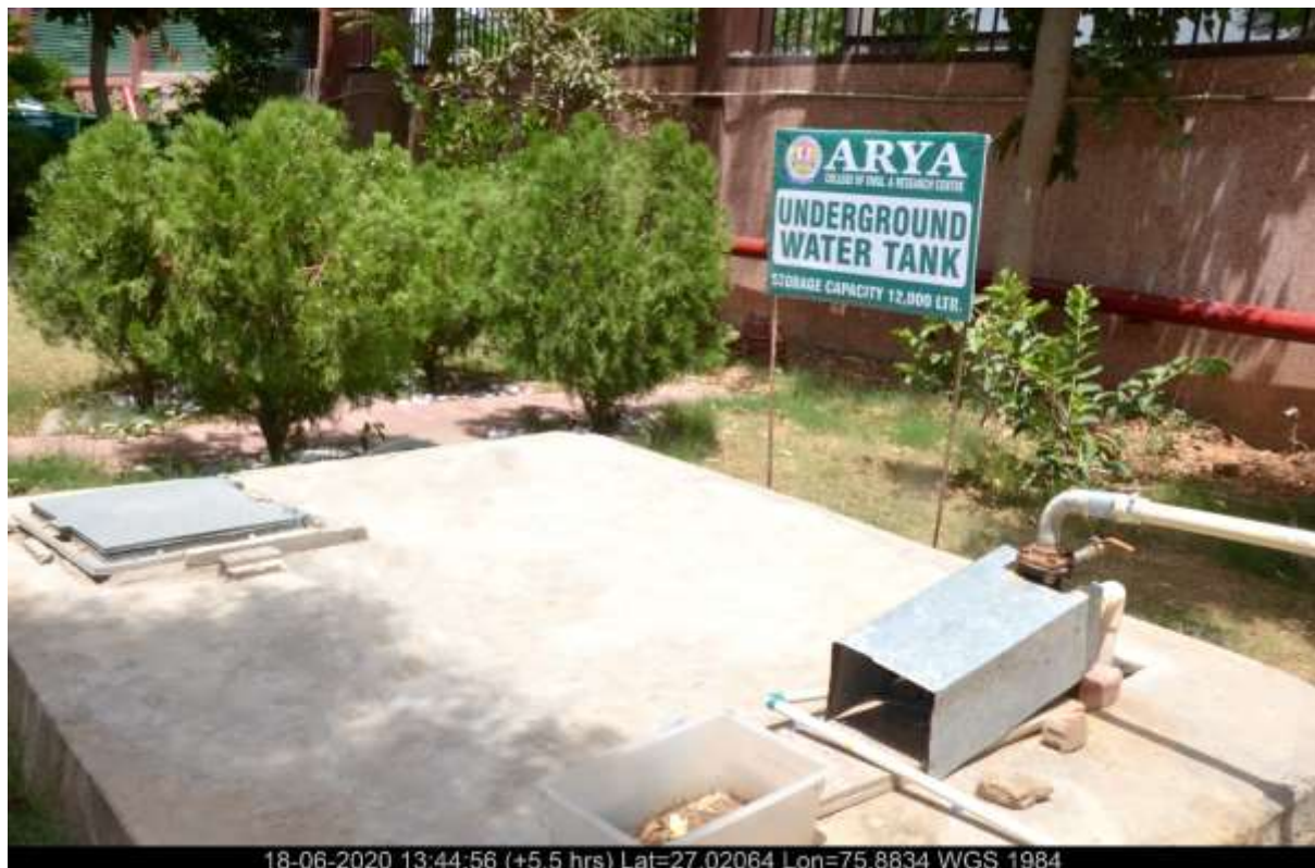
Underground Tank 2: Capacity 12,000 Ltr.
